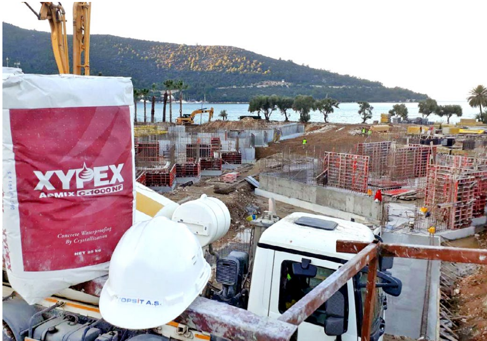
Construction adjacent to sea
